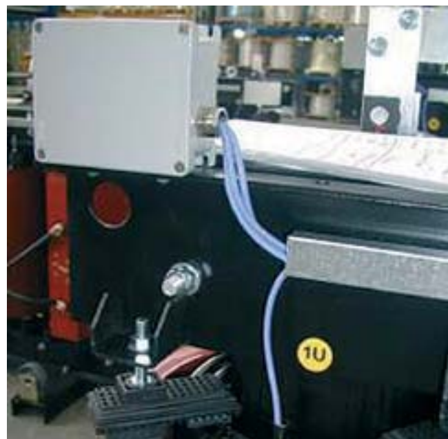
^ Example of installation of a Pt100 temperature control unit
